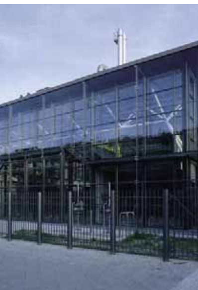
Abwasserpumpwerk Sewage pump station
