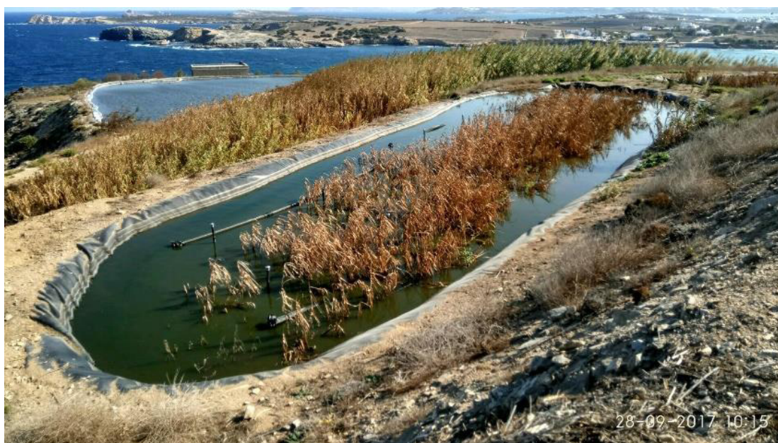
Figure 34 Dead local plants before rehabilitation actions in Antiparos WWTP due to clogging of top layer.
