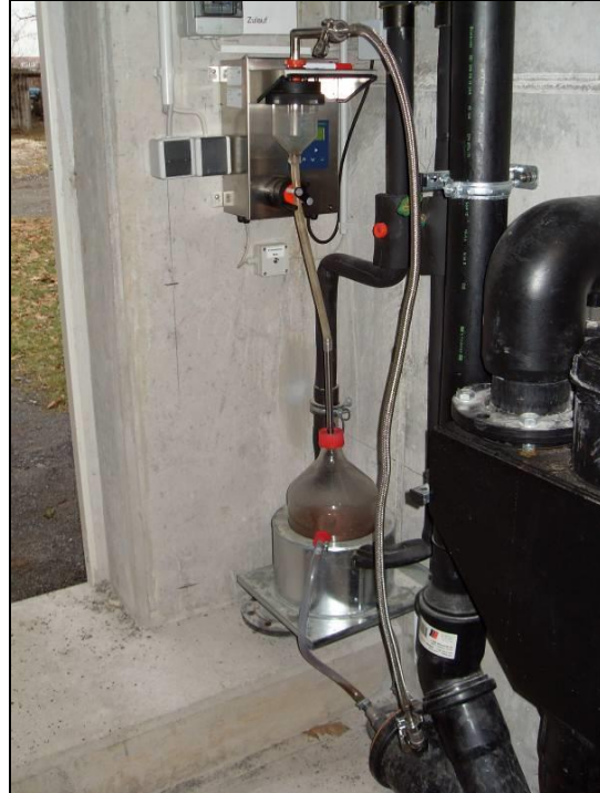
Figure 44: Influent sampling system at the BDZ (COMPAS)
