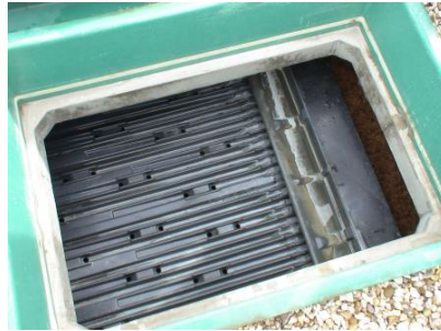
Figure 28: Distribution plate assembly – Ecofix® biofilter
