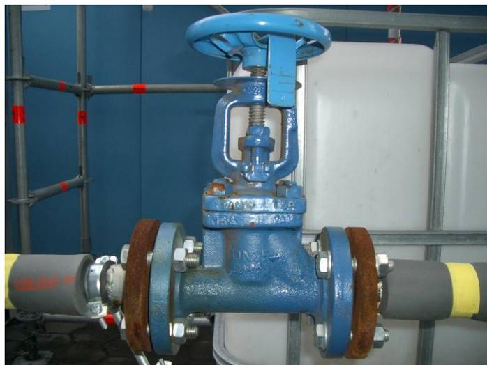
**Picture 8:** Steam valve of steam stripping plant in demo-size
