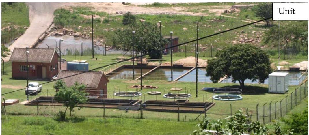
Figure 2 - The pilot unit at the test location in Ogunjini, South Africa
