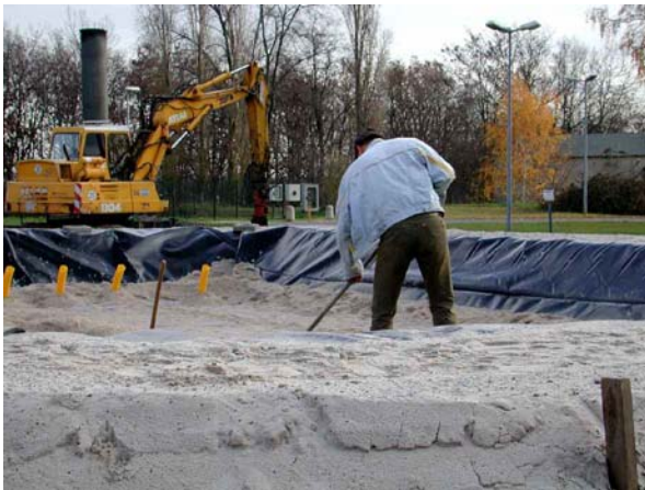
Realisation of constructed wetland (status: 24.11.03)
