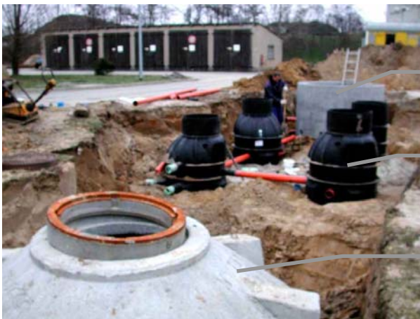
Unit operations of constructed wetland (status: 8.12.03)
