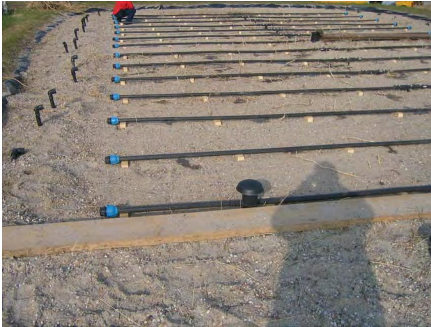
**Fig. 2.4.18:** Constructed wetland, distribution system
