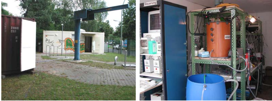
Figure 7. Site (Grünau pumping station) and pilot unit of preliminary study
