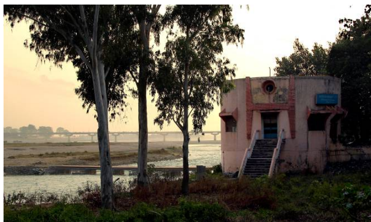
Fig. 2-2 Example of a large-diameter RBF well adjacent to the Ganga River in Haridwar (Photo: L. Rossoff, HTWD, 2011)
