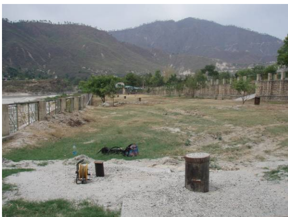
Fig. 4-3 Monitoring well MW4 (left) constructed in Srinagar in between PW4 (right) and the Alaknanda (Photo: K. Heinze, HTWD, May2012)
