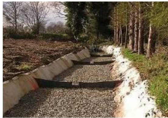
Figure 10: View of the ditch (towards inflow) with barriers.
