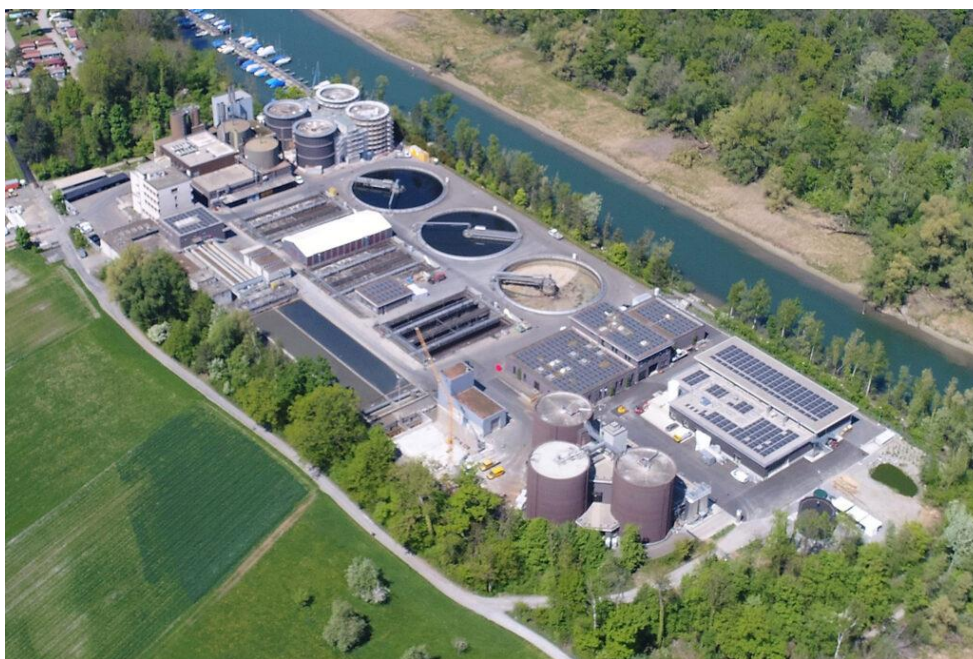
Figure 2: Aerial view of WWTP Altenrhein
