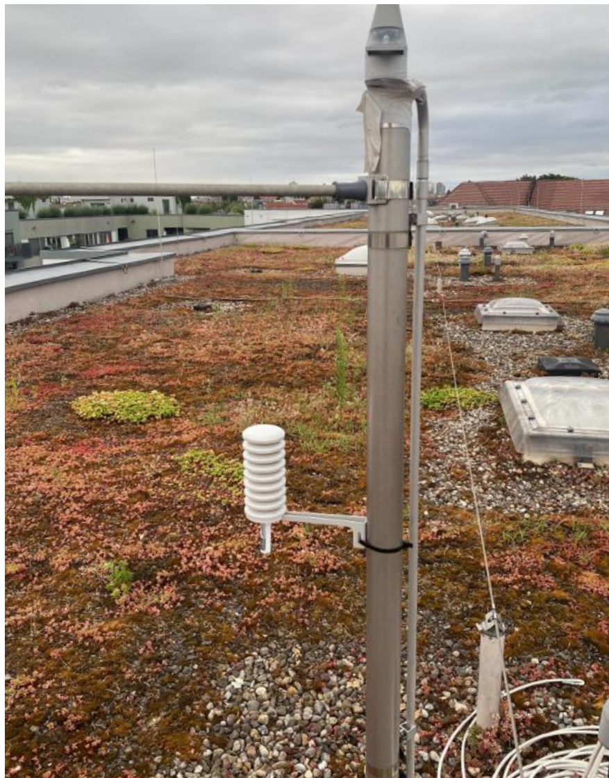
LoRaWAN temperature sensor on an extensive green roof
