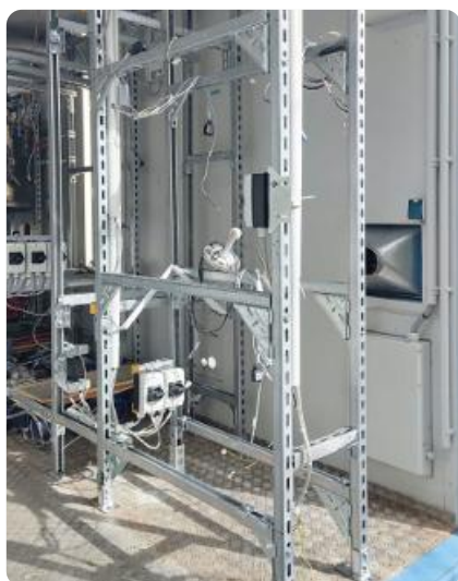
Re-erection of the assembly scaffolding
