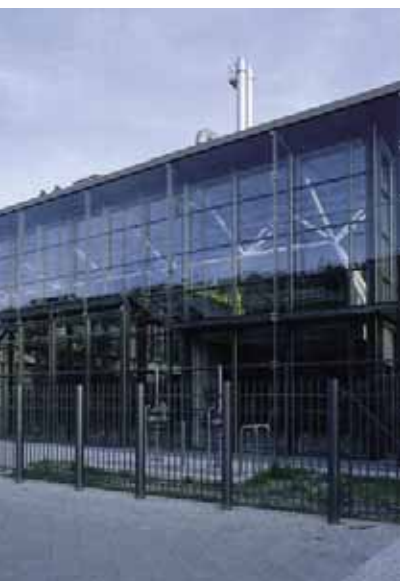
Abwasserpumpwerk Sewage pump station
